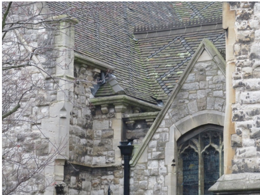
Complicated area of rainwater disposal adjoining the north transept.
